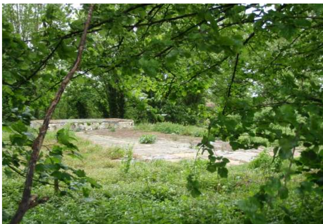
Plate 2. View of looking north and showing demolished building foundations
